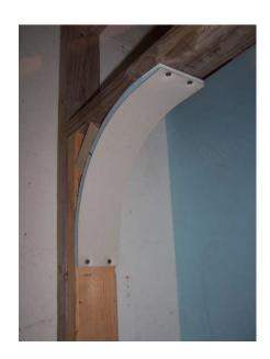
Fasten corners in place with drywall screws
