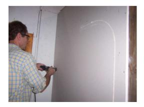
Install face-sheet, roto-zip opening. Screw into blocking
